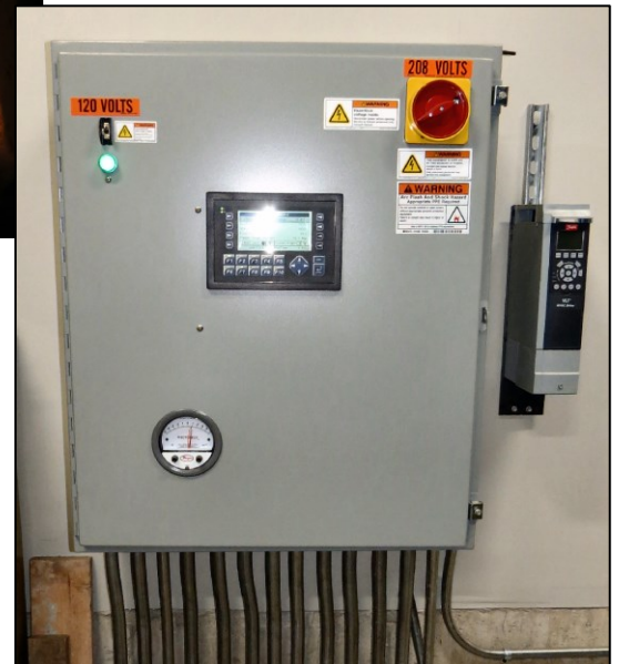
Computer software controls the entire heating system. Warnings can be received remotely.
