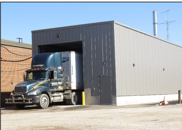
Heating plant and chip storage building, next to school.
