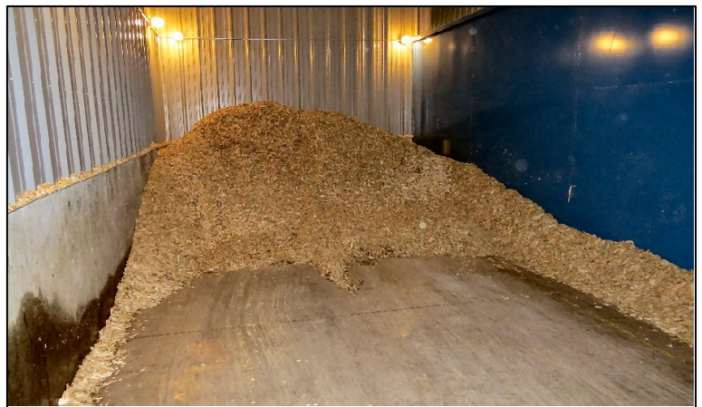
Wood chips inside storage bin. Walking auger underneath chips.
