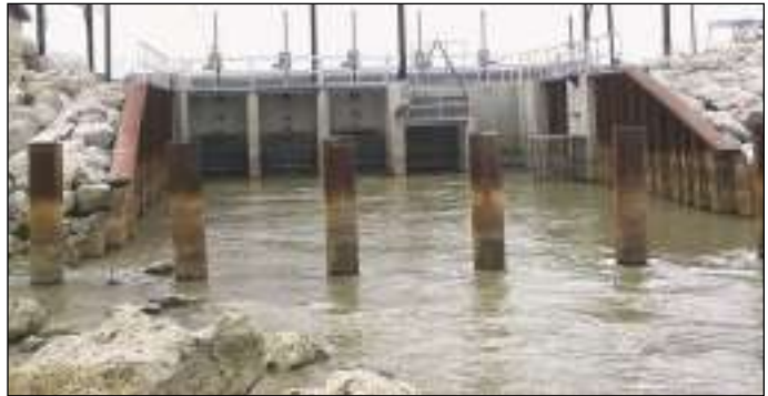
Metzger Marsh. Five large gates provide effective control of the water levels in the marsh, while grates control entry of large fish.
