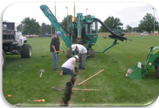
Left: Cutting drain lines and installing drain tiles, Intramural Field, Michigan State University, East Lansing, Michigan, July 200.
