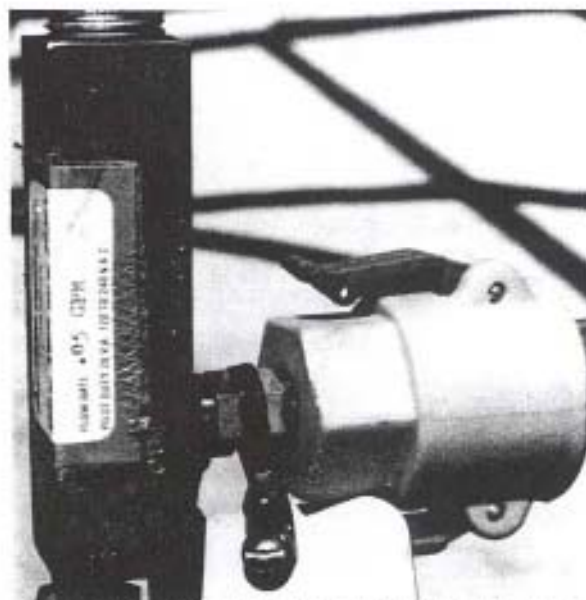
A flow sensor on the chemical injection line can shut down the irrigation system and pumping plant if chemical flow stops.
