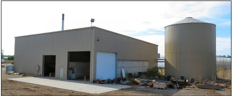
Power plant and 210,000-gallon thermal storage tank.
