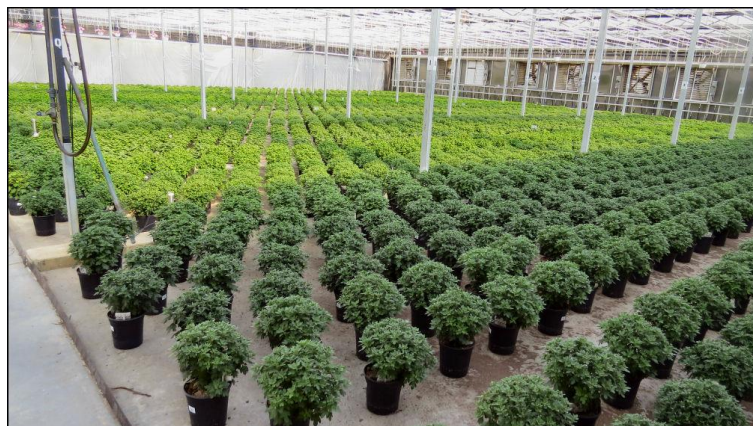
One of the greenhouses heated with wood chips.
